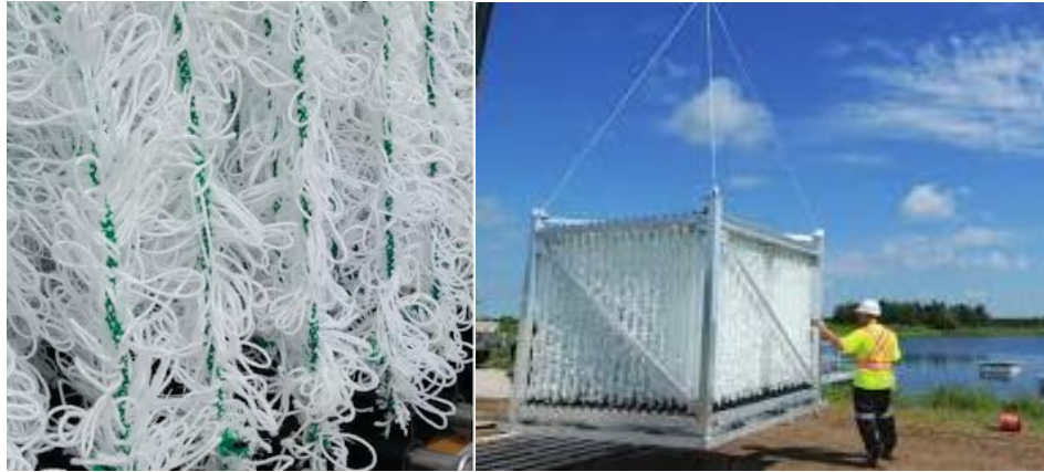
Figure 10-1: BioCord® installation (Courtesy of Bishop Water)
