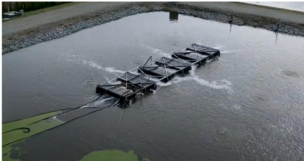
Figure 10-2: Ecofixe in Lagoons (Courtesy of Technologies Ecofixe)
