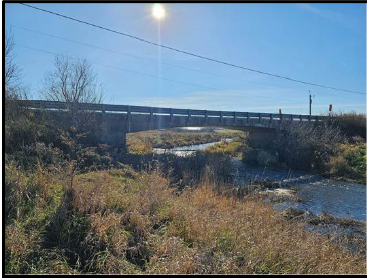
Roxborough - Finch Boundary Culvert (BCI = 50 Fair)
