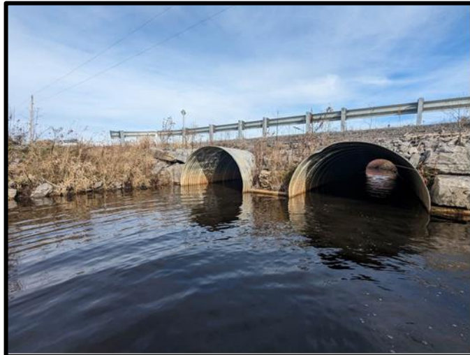
Bender Road Culvert (BCI = 75 Good)
