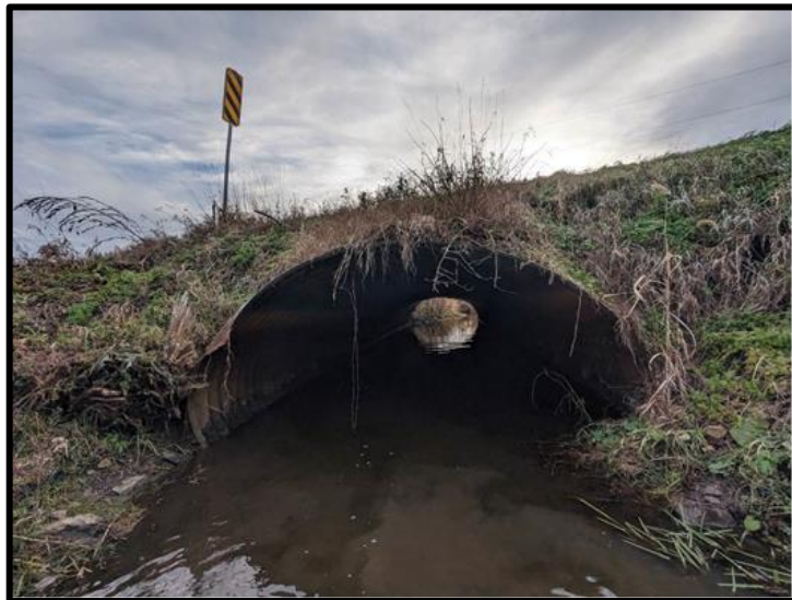
Roxborough - Finch Boundary Culvert (BCI = 50 Fair)
