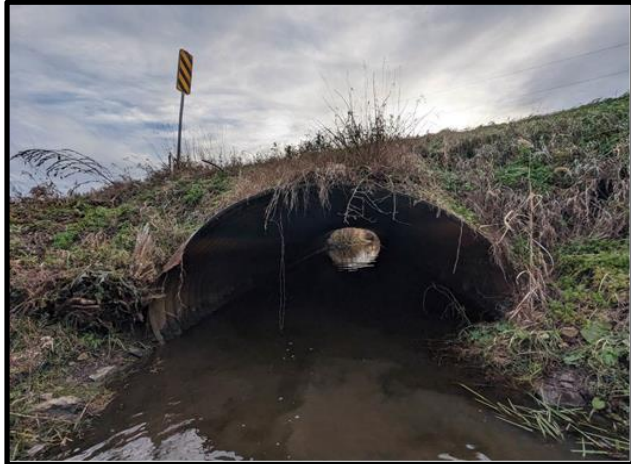
Roxborough - Finch Boundary Culvert (BCI = 50 Fair)
