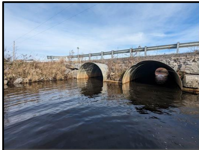
Bender Road Culvert (BCI = 75 Good)
