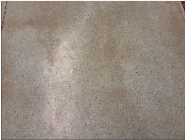
Non-asbestos vinyl sheet flooring with blue and white specks.
