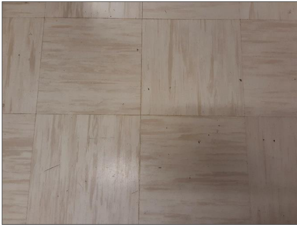
Non-asbestos vinyl floor tiles with large white and beige streaks.
