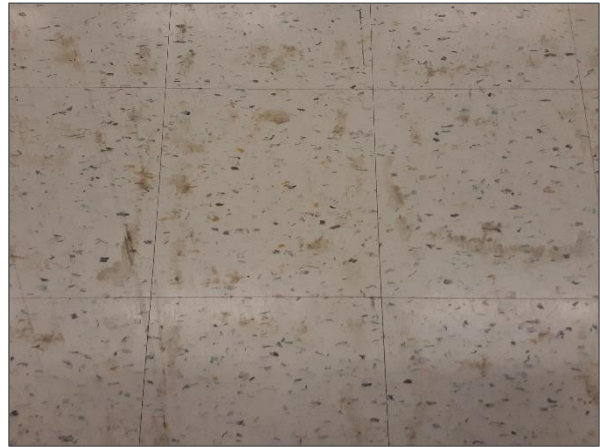
Non-asbestos vinyl floor tiles with large white and grey streaks.
