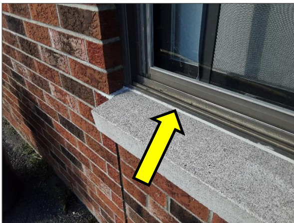
Non-asbestos light grey caulking.
