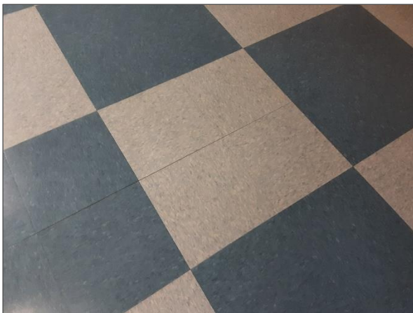
Non-asbestos blue and light blue vinyl floor tiles with fleck.
