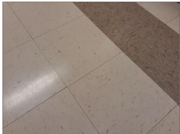
Non-asbestos grey and beige vinyl floor tiles with fleck.
