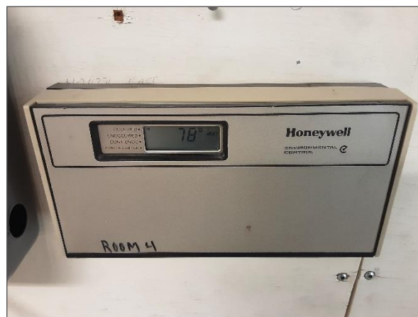
Non-mercury digital thermostat.
