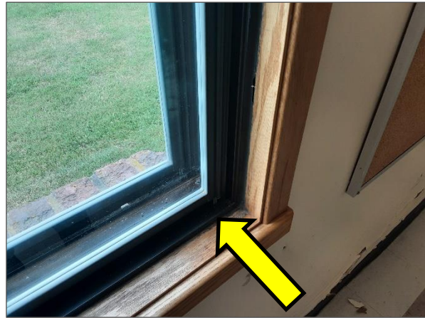
Non-asbestos dark brown caulking.
