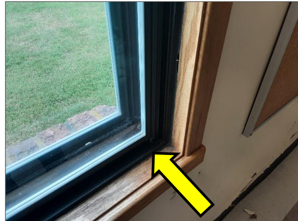
Non-asbestos dark brown caulking.
