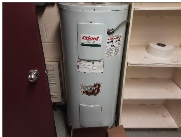
Hot water tank insulated with non-asbestos fibreglass.
