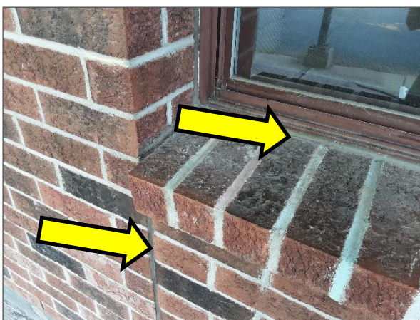
Non-asbestos light brown caulking.
