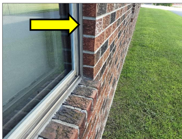
Non-asbestos brown caulking.
