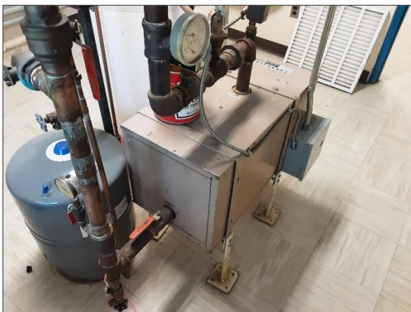
Furnace insulated with non-asbestos fibreglass.
