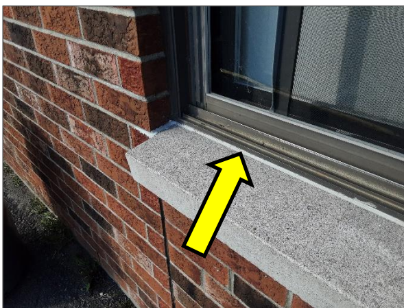
Non-asbestos light grey caulking.
