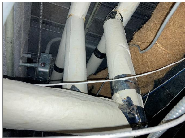
Pipes insulated with non-asbestos fiberglass.
