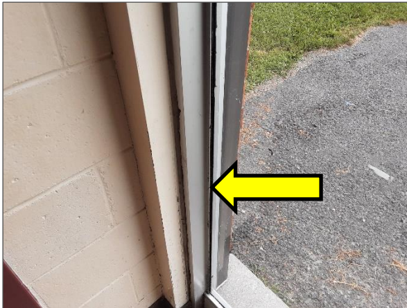
Non-asbestos black butyl sealant.
