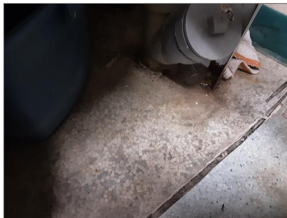
Non-asbestos vinyl sheet flooring with grey squares.
