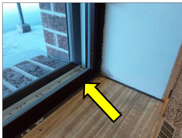
Asbestos-containing hard brown caulking.
