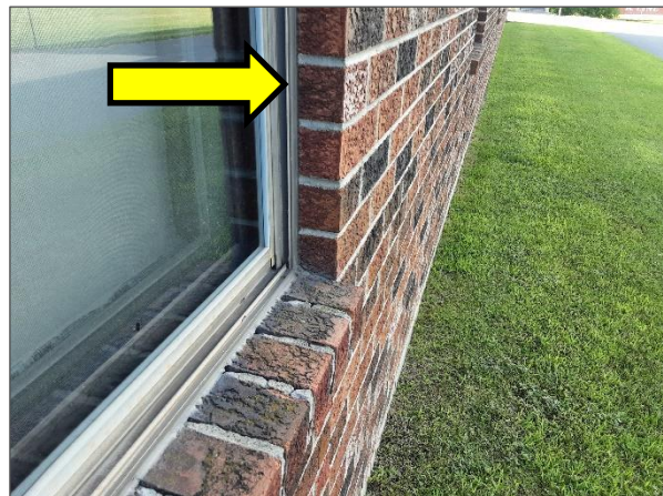
Non-asbestos brown caulking.
