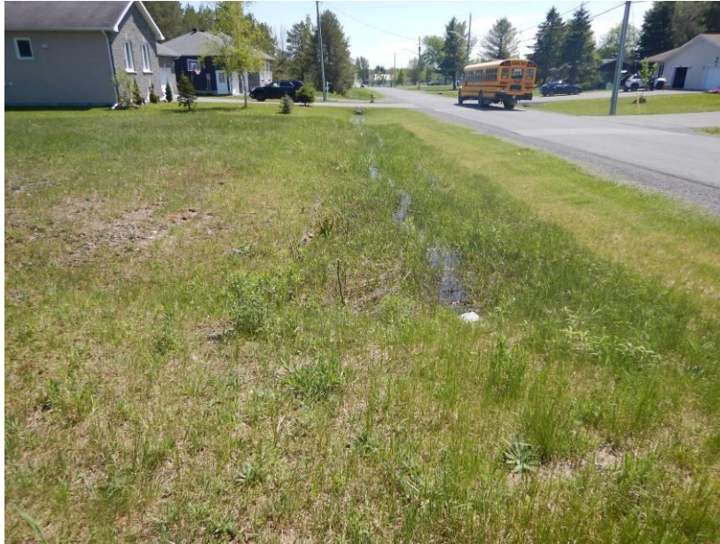
Photo 5: Portions of the Tributary Running along Valley Road (May 18, 2022)
