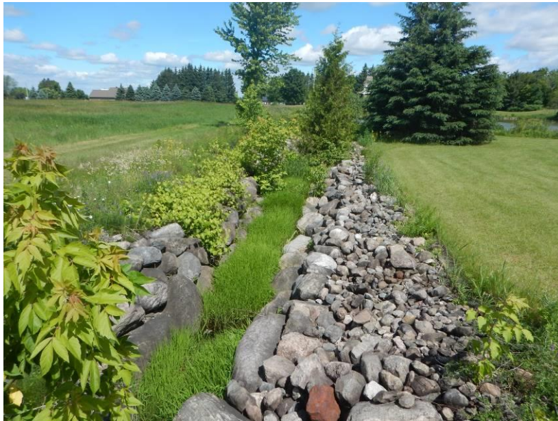
Photo 17: Pond Outlet (June 13, 2022)
