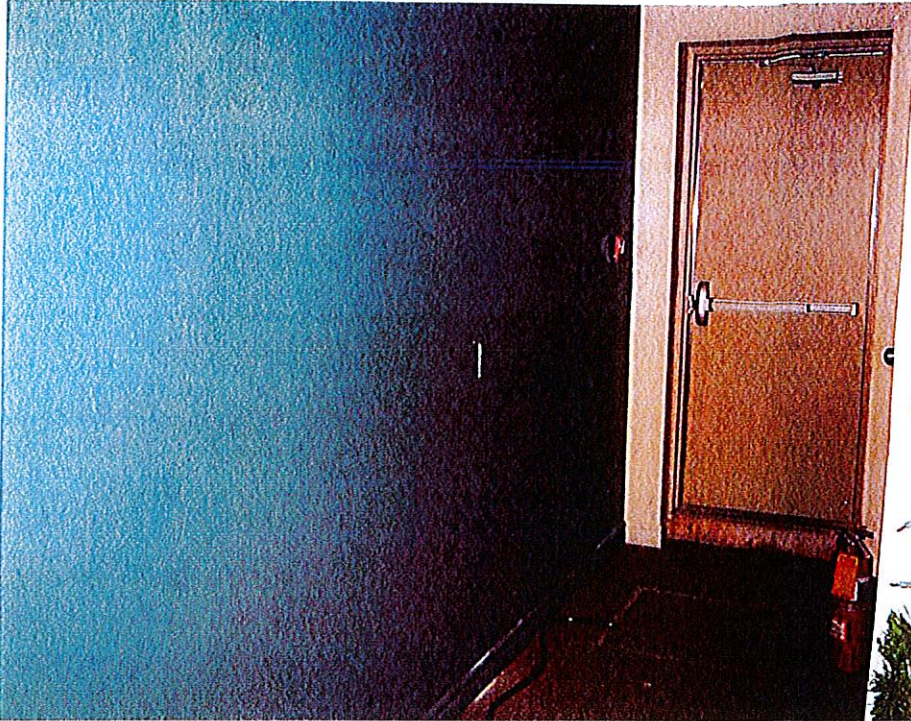
Photo 3: Location of samples S7, S8 and S9 (drywall in basement) for asbestos testing. This material did not contain asbestos.
