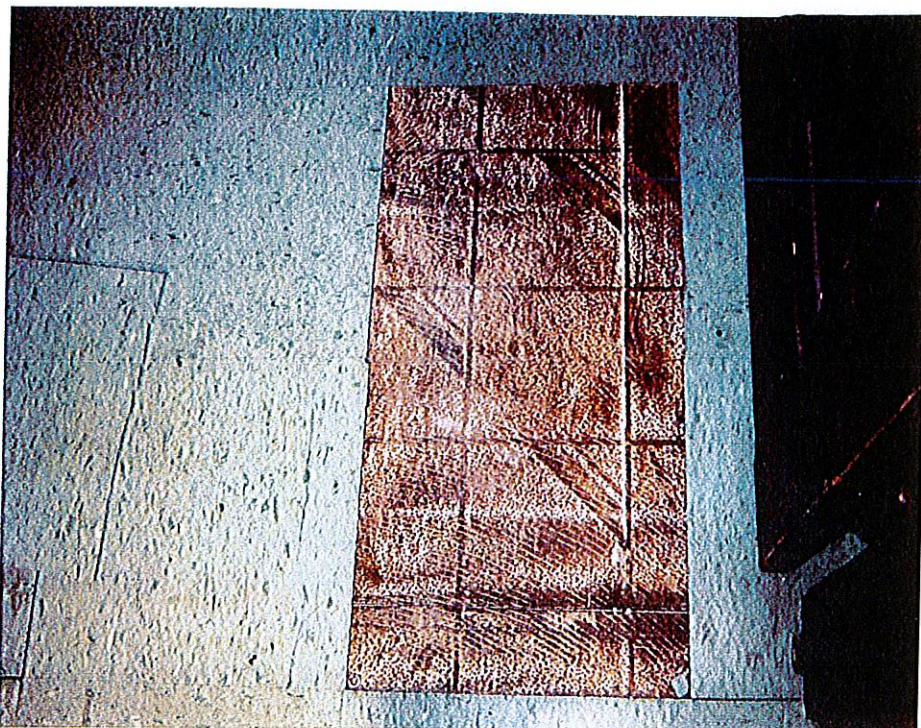
Photo 7: Location of samples S13, S14 and S15 (green, floor tiles, 2 nd floor) and S28, S29 & S30 (vinyl sheet flooring) for asbestos testing. This material did not contain asbestos.
